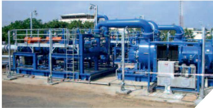
In order to overcome the high backpressure of the pipeline which constraints productivity of the well at offshore, the Multiphase Pumps were installed at the onshore terminal.
